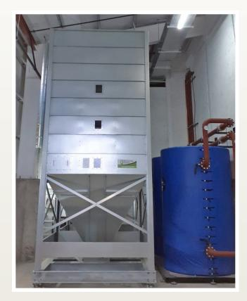
The silo itself was installed inside a basement and was not usually visible so we supplied a weigh cell system to give constant communication of the current fuel level to a building management system to ensure that the silo will never run out of fuel. In order to install the weigh cell system a galvanised mounting frame was manufactured and the silo was built on top of the frame.
