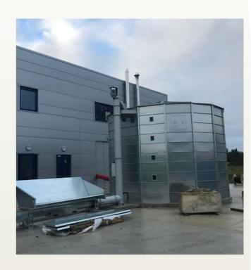
We installed a 90m3 wood chip silo made from galvanised steel and a loading auger capable of transporting wood chip from a tipper truck into the silo at a speed of 45m3 per hour.
