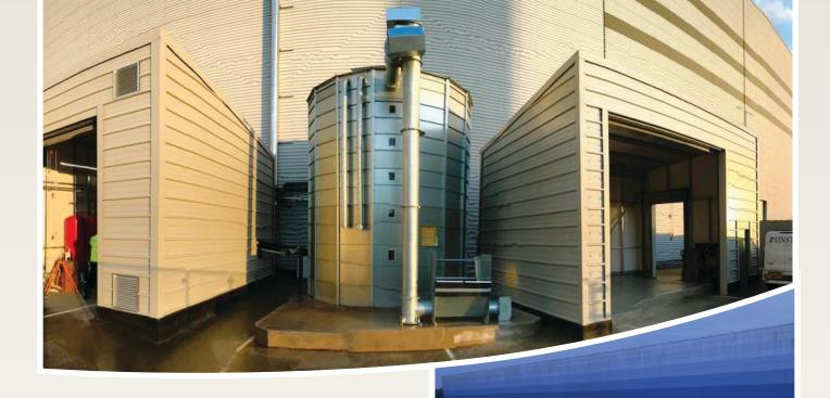
The 90m3 capacity silo was also fitted with fill and vent pipework to allow for blown deliveries of standard wood chips for times when the heat demand outstrips the availability of shredded timber.
